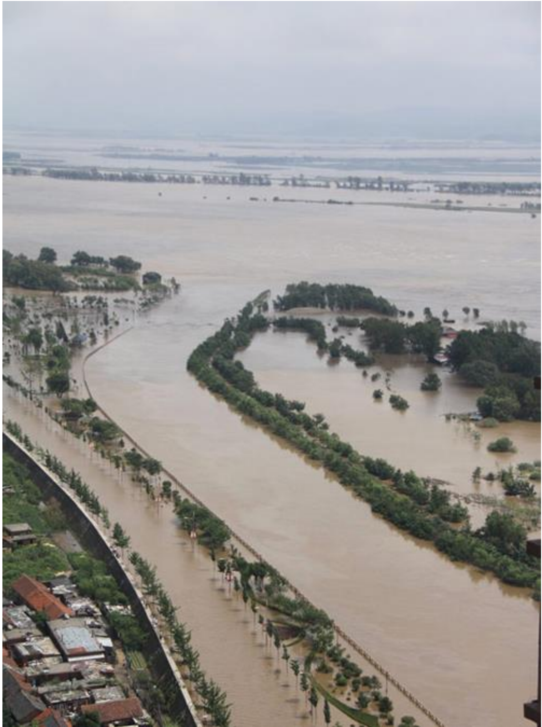
Figure 2-3 Yanjiang road was flooded on August 21 st , 2010
