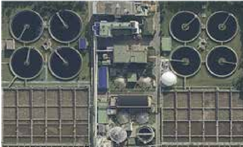
Figure 3.10 Image of a Public Sewage Treatment Plant and Mimetic Diagram of the Sewage Treatment Process.
