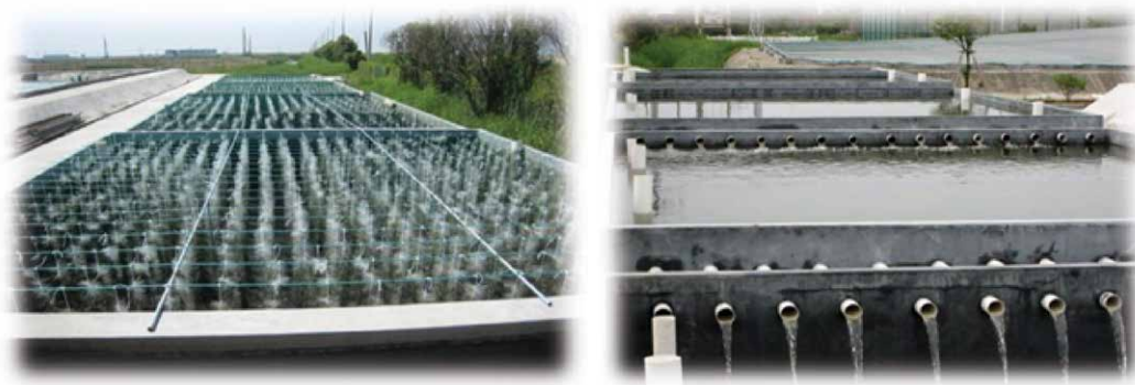
Figure 3-16 The quadruple tandem farming discharged water sedimentation tank in the discharged water treatment system. (Zhejiang Mariculture Research Institute)
